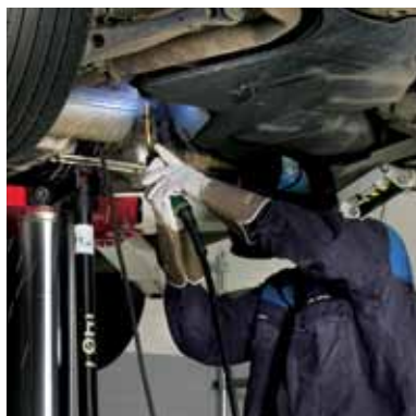
Repair of exhaust pipe suspension
